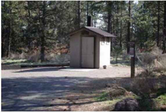
Figure 3: Typical single vault toilet
